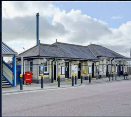
TRAIN STATION (CLOSEST) St. Neots Station
