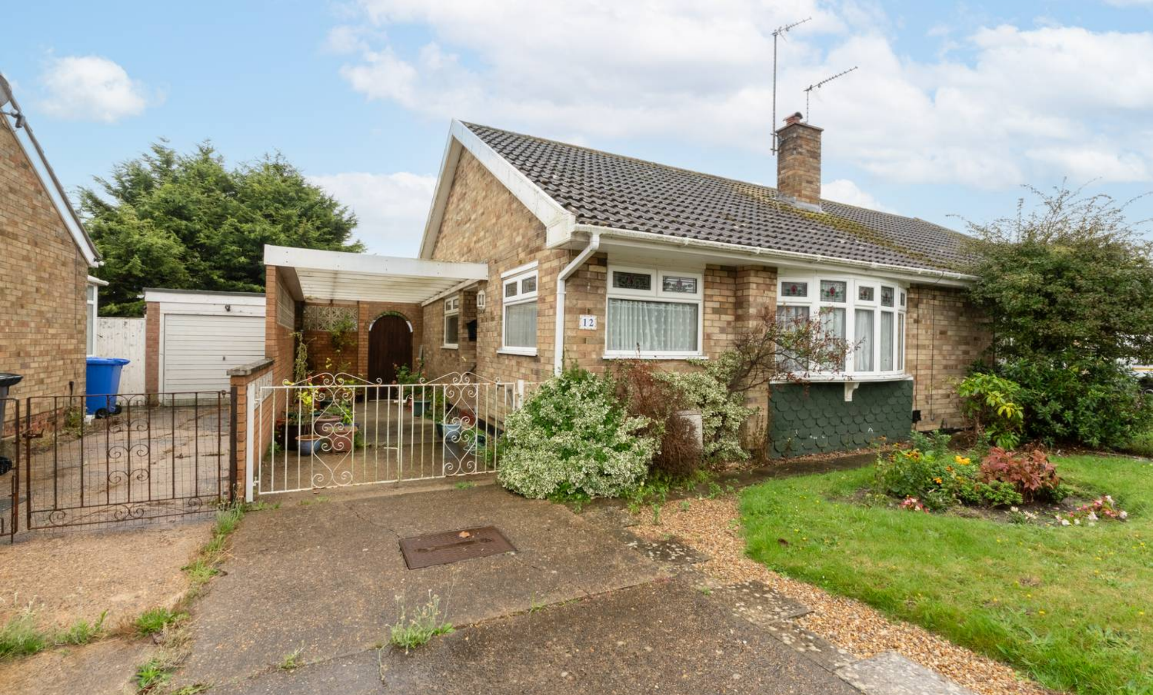
12 Fenlands Crescent, Lowestoft £200,000
