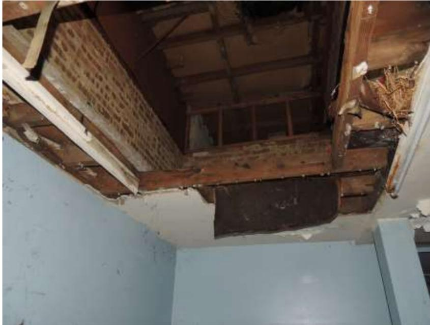
Damaged ceilings to the existing first floor and exposed second floor above
