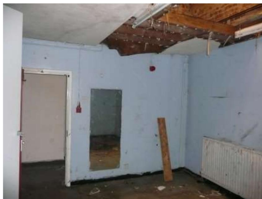
Internal spaces are generally in a very poor condition and appear structurally unstable
