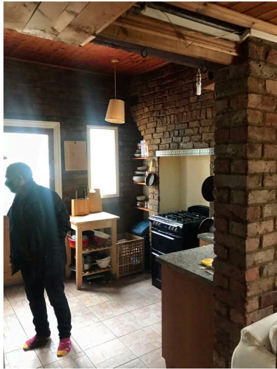
Figure 13 - dark interior (current kitchen)
