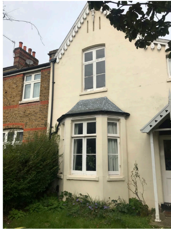
Figure 16 - Existing front of property Bay window which matches the terrace
