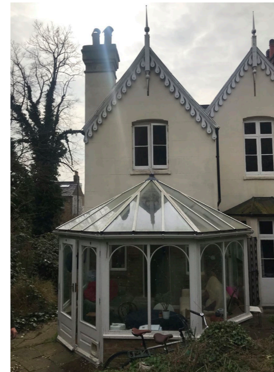
Figure 15 -Rear elevation showing traditional pitches and conservatory
