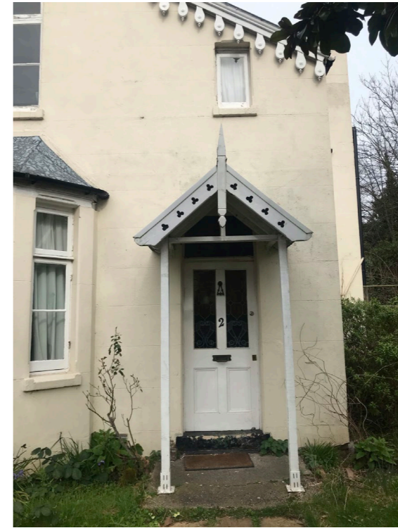
Figure 17 - Existing traditional looking porch
