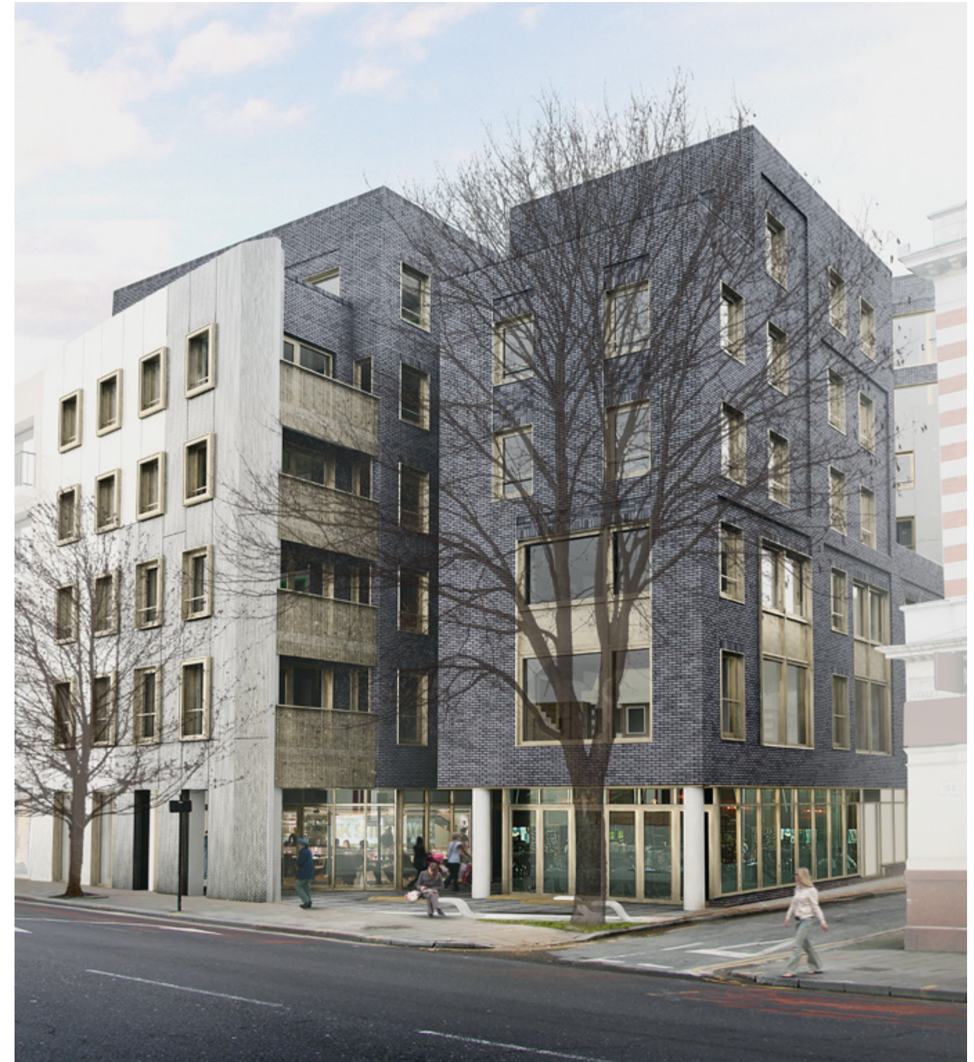
Monohaus, Mare Street entrance
