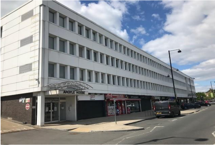
ARGYLE HOUSE, SUITE 1B, NORTH BLOCK, JOEL STREET, NORTHWOOD HILLS, HA6 1NW
